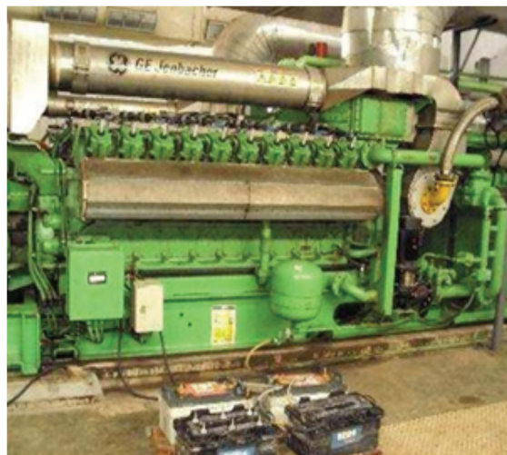
GE Jenbacher Gas Engine - Model J 320
