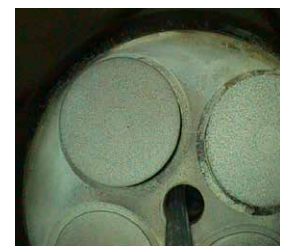
Figure 3 Valve deck ash layer
