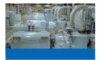
as impact servo valve operation and promote system foaming. Turbine systems are subject to contamination from several sources and deposits will accumulate even though the oil is clean. Inspect the system frequently and maintain the filtration system to its maximum effectiveness. Consult your OEM for their recommended ISO Cleanliness Level (also called ISO Particle Count).
